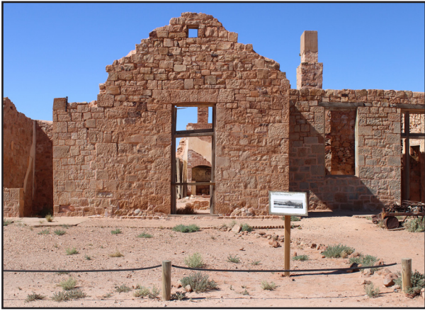
THE TRANSCONTINENTAL HOTEL AT FARINA. There are no longer any permanent inhabitants of the town but it has attracted volunteers from a wider region whose efforts have been to stabilise the remains. JLW.
