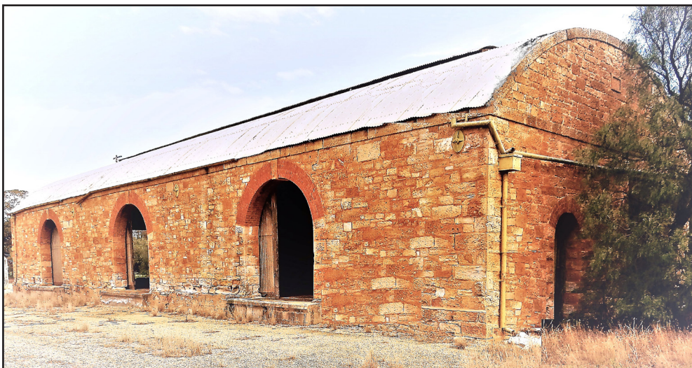
THE GOODS SHED AT HOYLETON. At the time this was built it was the only building of any substance at Hoyleton. The Wesleyans used it for their church services. It still stands but despite being heritage listed and the recipient of some restoration funding in 1988 it is still showing neglect. JLW.
