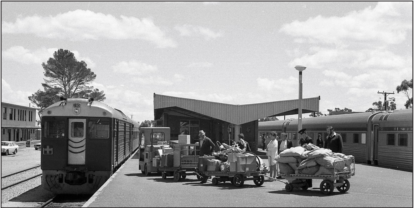
CHANGING TRAINS AT PETERBOROUGH. The train on the far track is the westbound Indian Pacific which has unloaded many mail bags that would have been from Broken Hill. On the near track is the Bluebird railcar, on the broad-gauge, that will travel to Adelaide via Terowie. When they constructed the Peterborough platform they gave themselves plenty of room. Quite different to the platform at Terowie. JLW.
