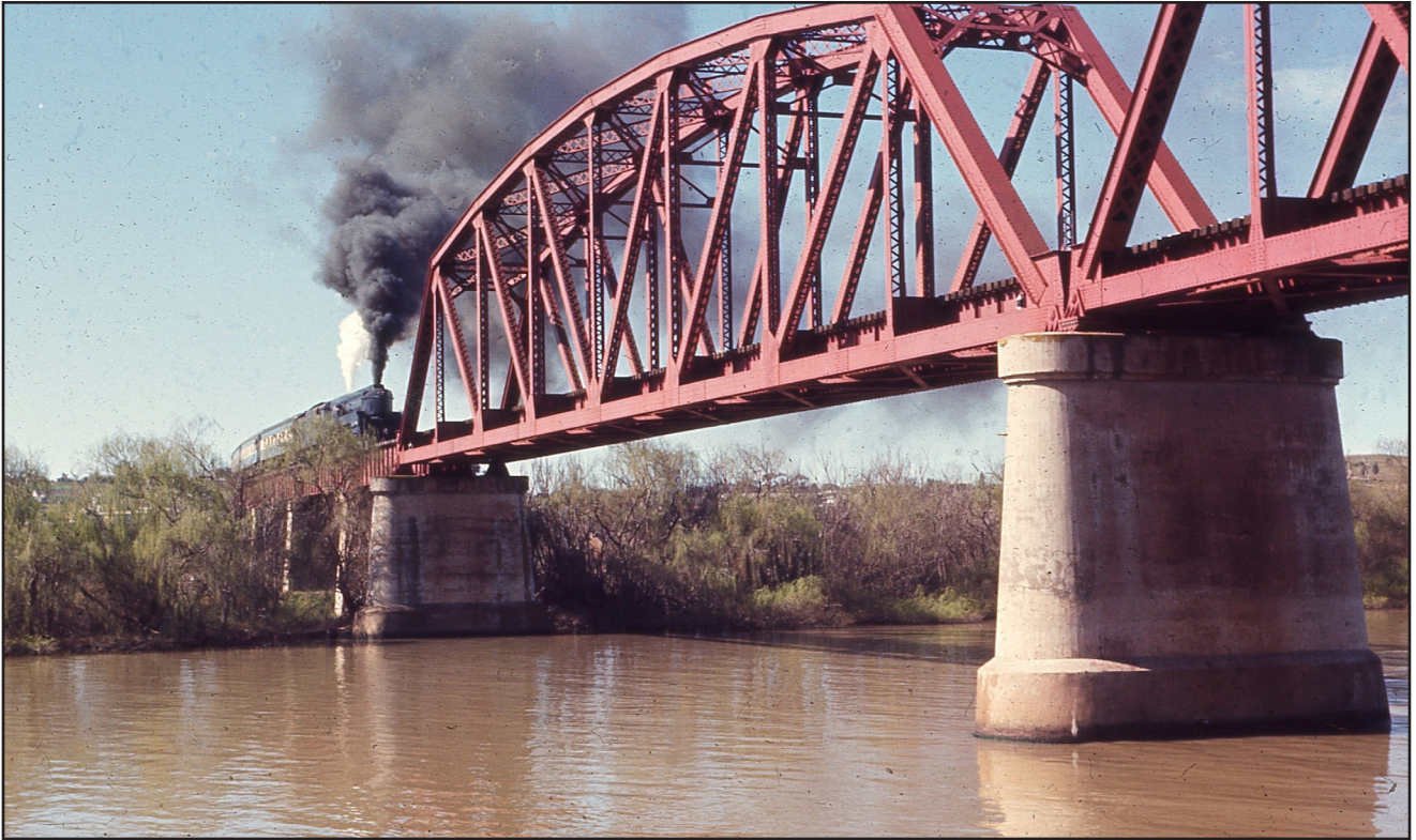
THE MURRAY BRIDGE, built in 1925, and made necessary by the progressive stressing of the original bridge and the impending arrival of the big engines. It was the most demanding single construction of many works carried out in South Australia in the 1920s as part of Chief Commissioner Webb's rehabilitation. The photograph features locomotive 526, with an ARHS special. JLW.
