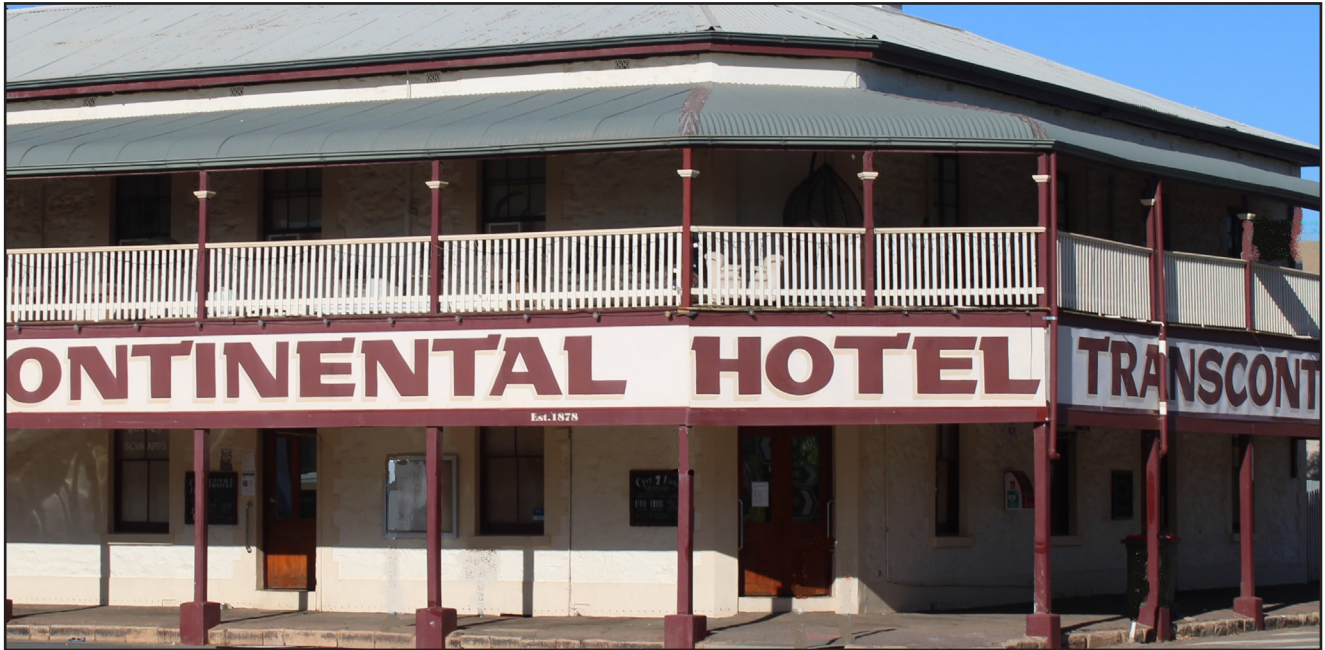
A TANGIBLE CONNECTION TO THE TRANSCONTINENTAL RAILWAY. At Quorn. The sign on the verandah is Est.1878. That was the year the Governor turned the first sod of the railway. JLW.
