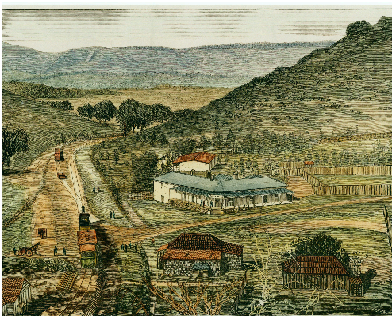
VIEWS ON THE PORT AUGUSTA AND GOVERNMENT GUMS RAILWAY, SOUTH AUSTRALIA: No. 1, SALTIA TOWNSHIP.
